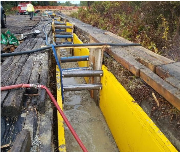
Fig 1: Dewatering trench at Frink farm, near Str. 106. Viewing west. (10-08-19).
