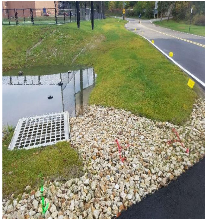
Fig 10: Rain garden at UNH, next to Colovos Rd. Viewing north. (10-08-19).
