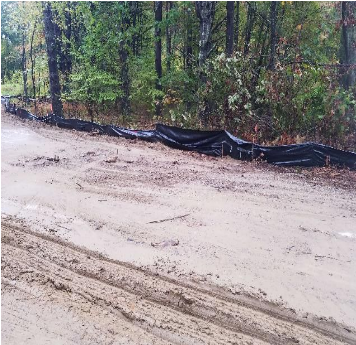
Fig 3: Silt fence installed along trench at Flynn pit. Viewing southeast. (10-08-19).
