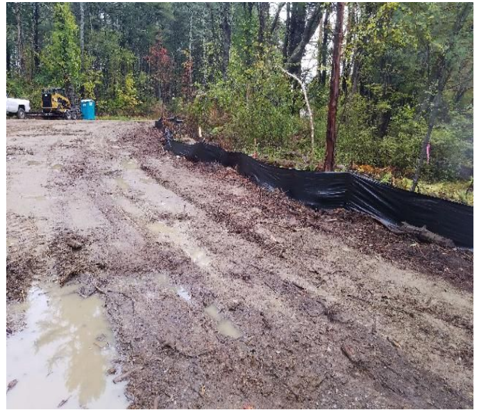
Fig 2: Silt fence installed along trench at Flynn pit. Viewing southeast. (10-08-19).
