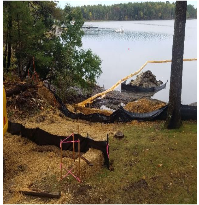
Fig 6: Sediment and erosion controls installed at the Beswick property. Viewing west. (10-08-19).
